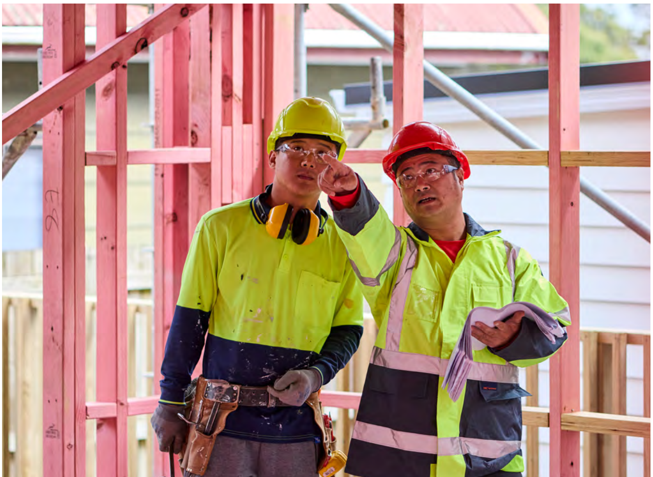
Building site, Auckland. Credit: Tanmay Desai, Truестock.
